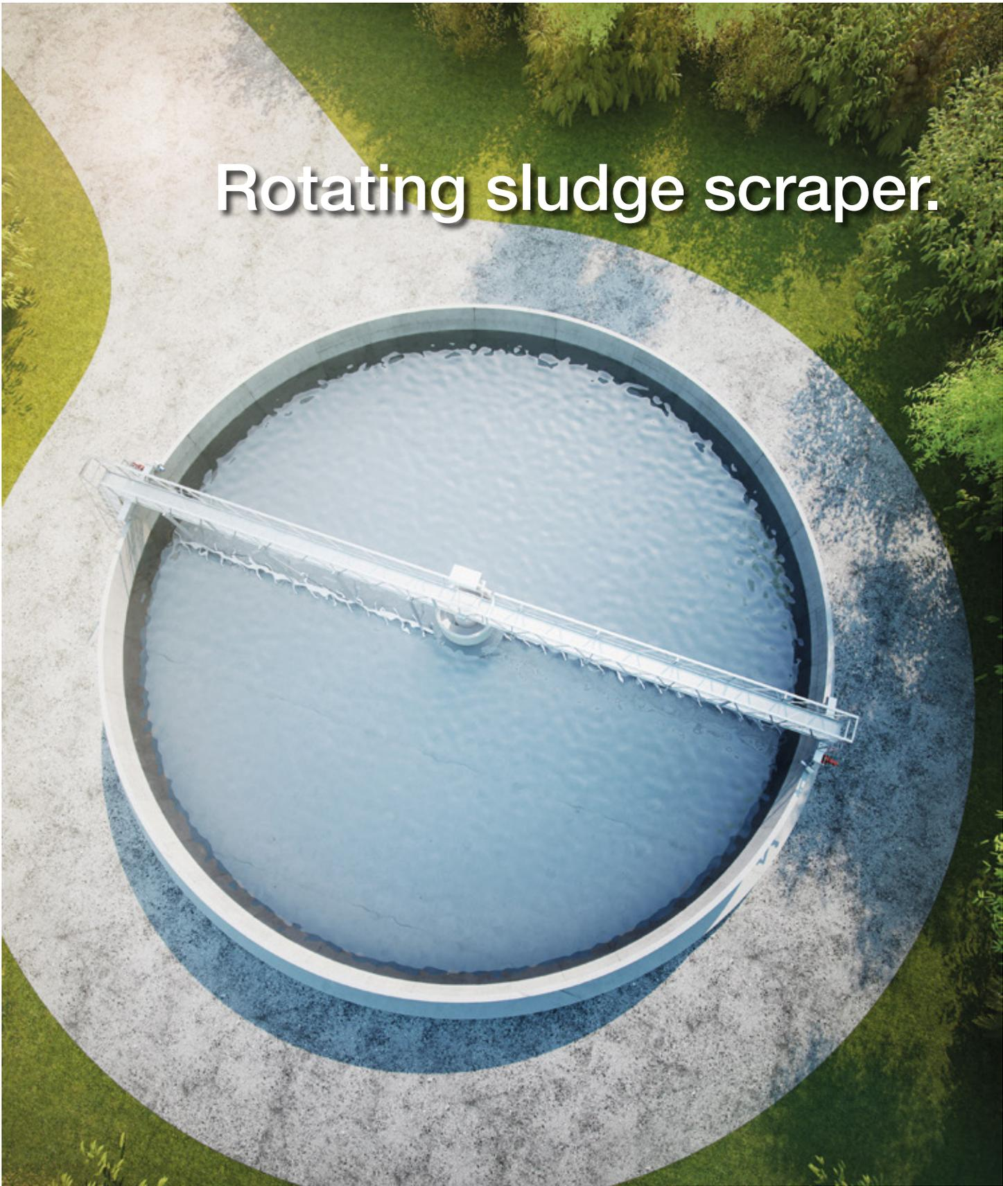
Sludge scrapers for circular tanks utilize either central drive or peripheral drive. This depends on the process, tank diameter, design and sludge loads.
